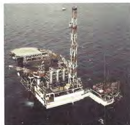
Figure 3 Cleeton Production and Wellhead Platforms
