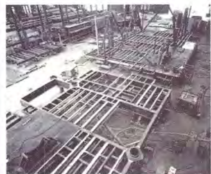
Figure 11 Topsides Steelwork As Built (15.6.95)
