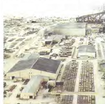
Figure 16 The "McDermott" Yard at Ardersier
