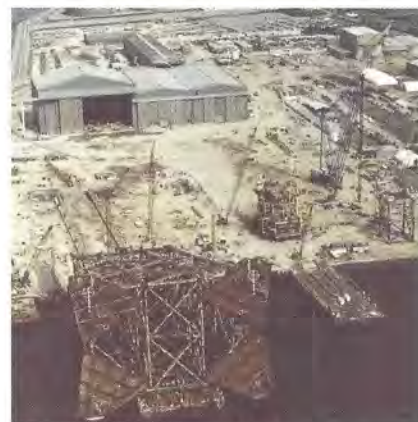
Figure 15 The "HIFAB" Yard at Nigg
